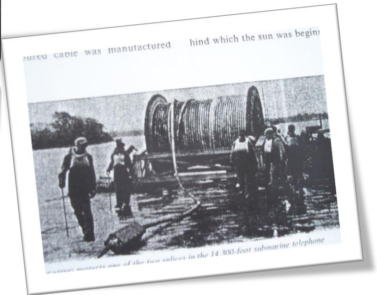
14,000 foot telephone cable, spinning out from barge
